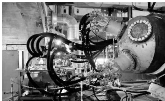
Fig. 9 Connection of a SG to the AMDA deployed by AREVA NP to apply the CORD process
