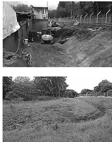
Fig. 4 Discharge channel under excavation work (upper), and after the remediation work (lower)
