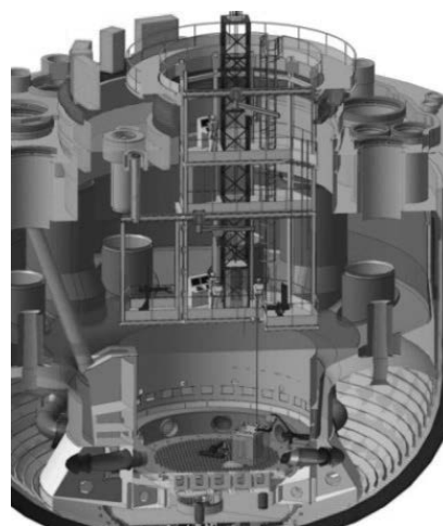
Fig. 16 Reactor vessel internals dismantling 23) (2017-2024)
