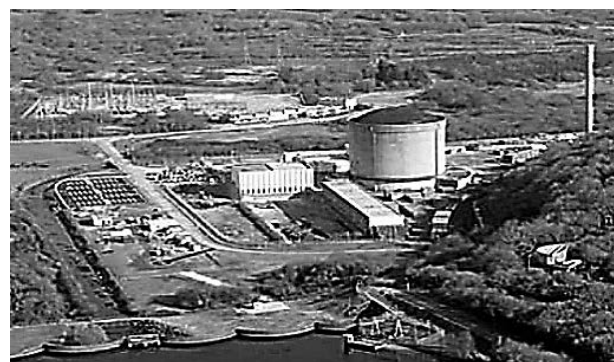
Fig. 3 Brennilis nuclear power station
