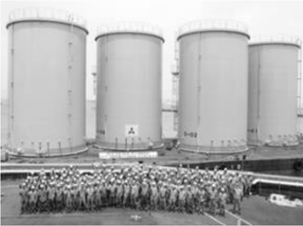
Fig. 22 Welded type liquid waste storage tank
