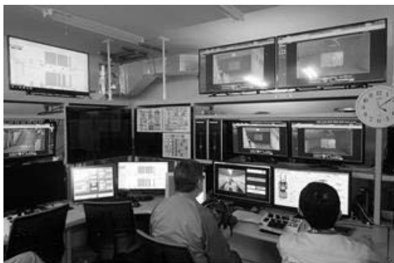
Fig. 19 Remote monitoring and control room
