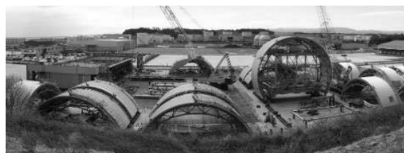
Fig. 15 Practice of cover construction in off-site yard
